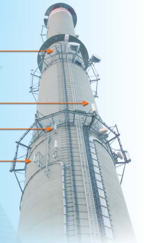
Multi-Operator Antennas
